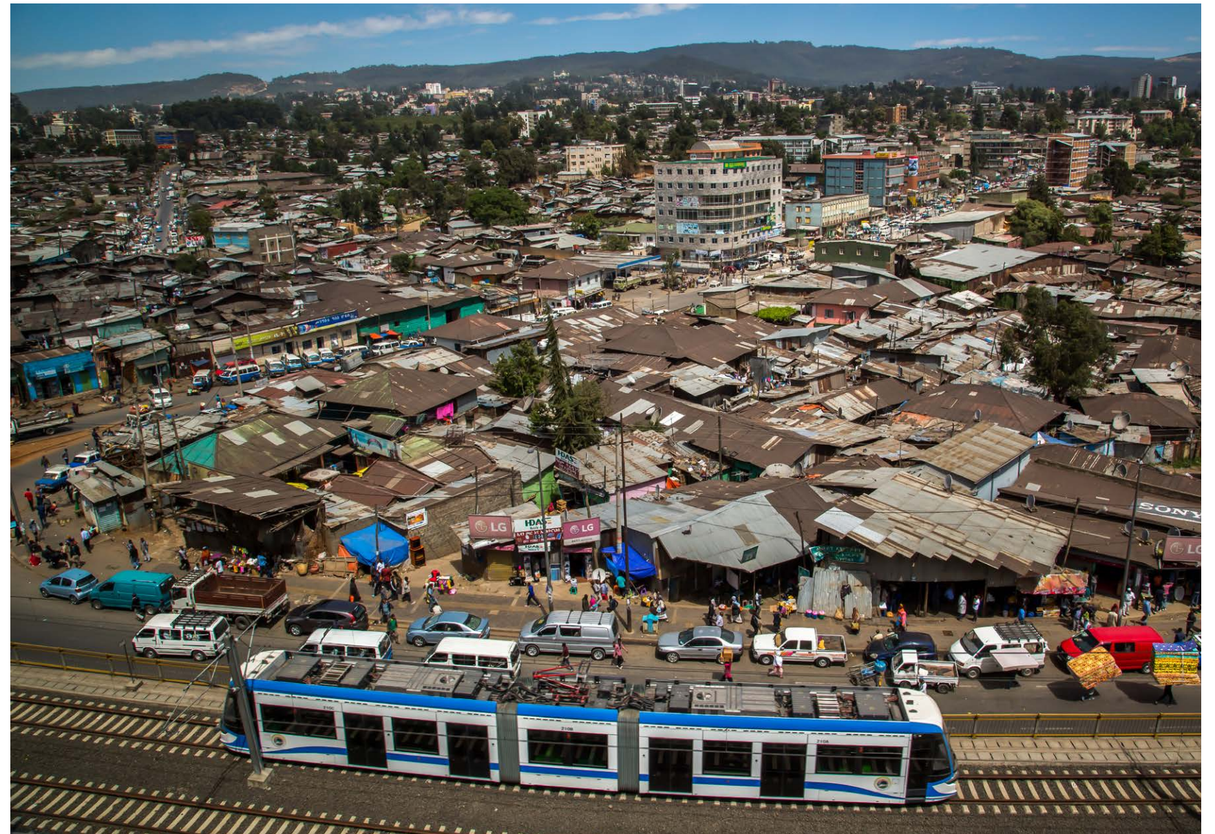
Light rail in Addis Ababa, Ethiopia, brings efficient and environmentally friendly transportation to the city.
